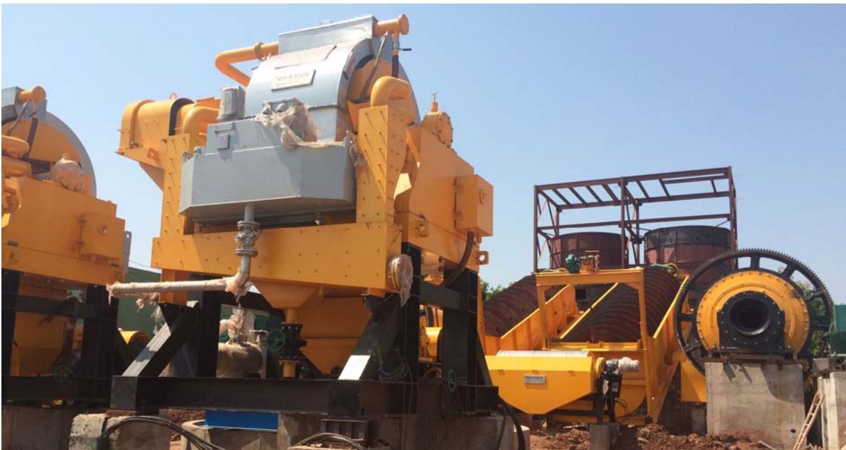
Final Fitout of Chinese Equipment
