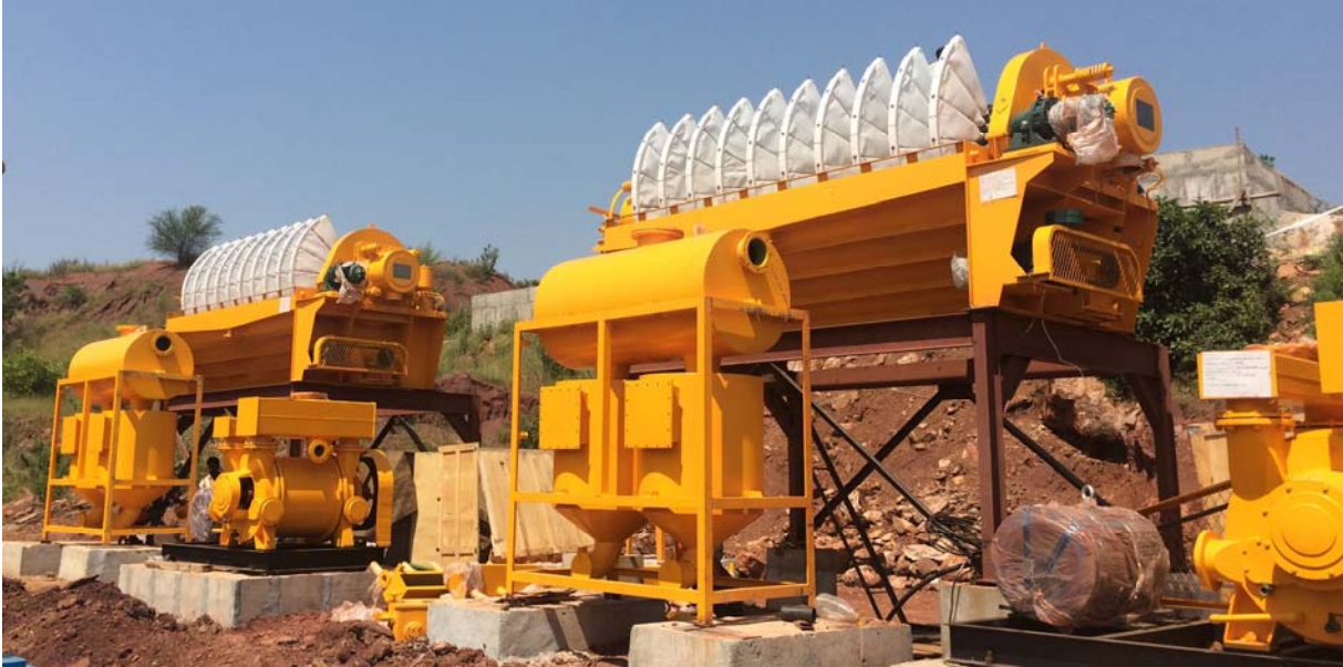
Final Fitout of Chinese Equipment
