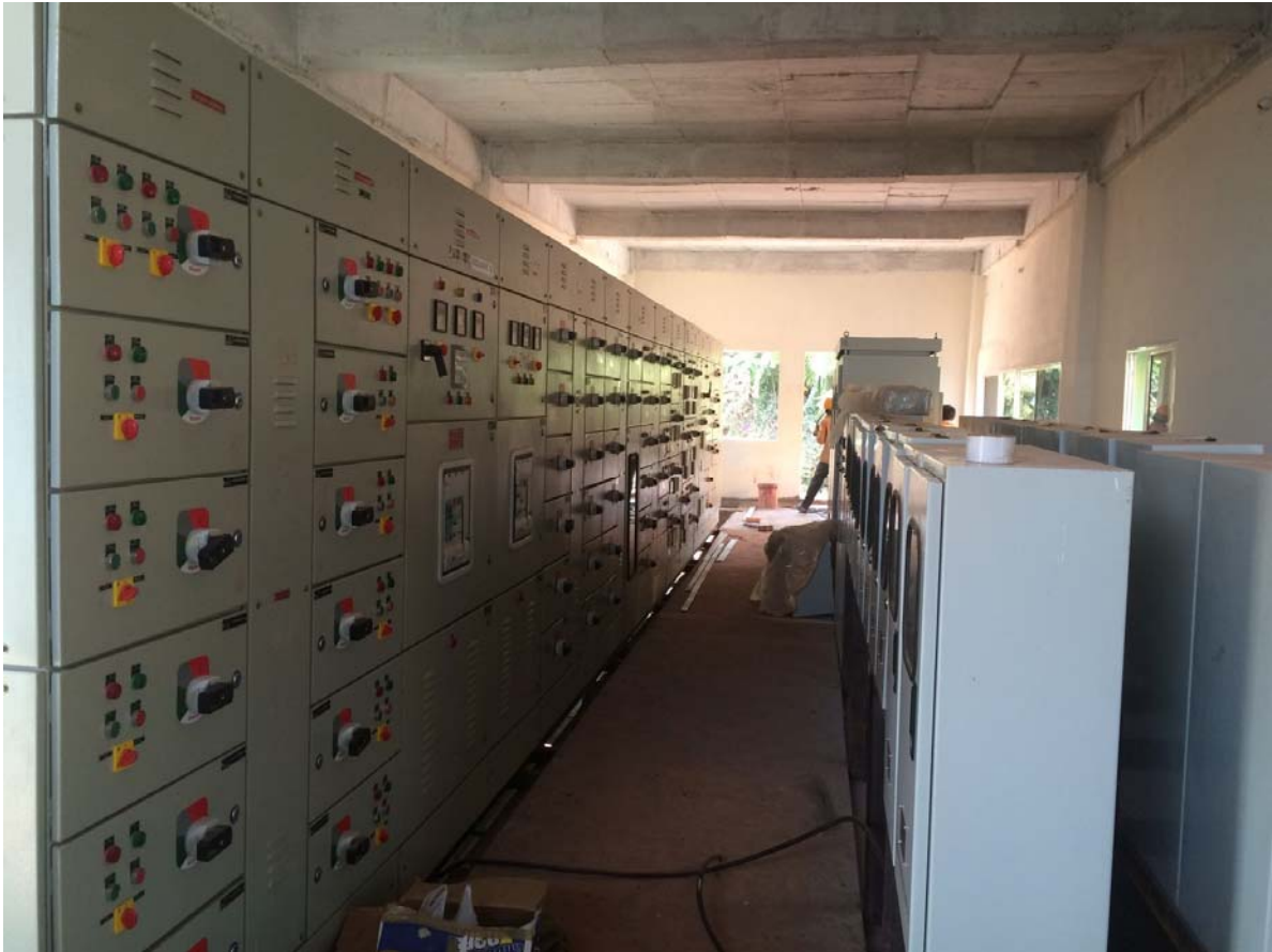
Internal Control Room Testing
