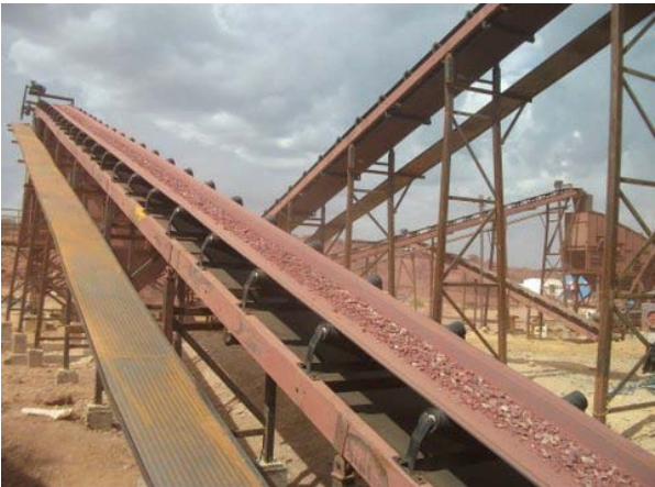
The existing NSL Phase One beneficiation plant:
