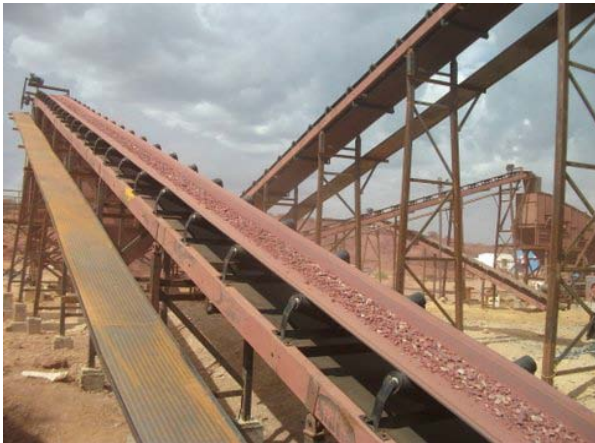
The existing NSL Phase One beneficiation plant:
